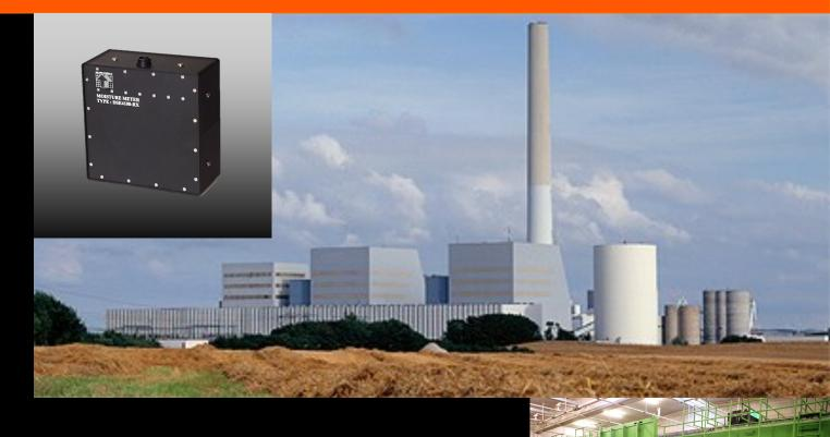
The other reason is their ability to control their own process. It is extremely important for a power plant to manage the combustion in their boilers and the only way, this is possible, is to know the content of moisture of the biofuel they are putting into the boilers. For a bioethanol plant, knowing the moisture of the straw, can increase their yield up to 5 %, meaning many tons of additional bioethanol produced, that otherwise could go lost.
